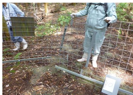
侵入防止柵の点検
