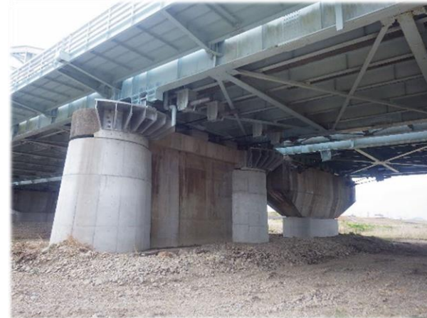
橋梁の耐震補強
