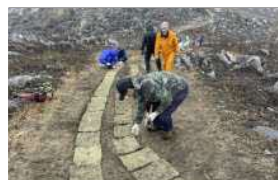
歩道の補修作業 Trail Maintenance
