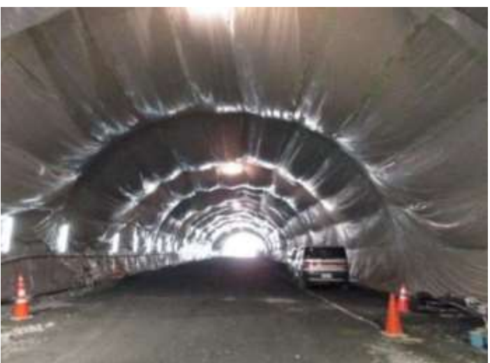
Picture of curing after form removal
